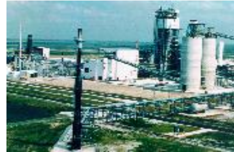
Tampa Electric 250-MW IGCC Power Plant
