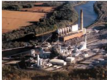
PSI Energy Wabash River 300-MW IGCC Power Plant
